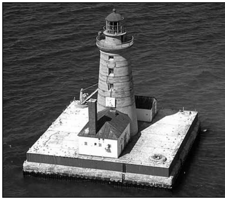
LOCATED in a lonely spot in northern Lake Huron, the robust design of the Spectacle Reef Lighthouse, completed in 1874, set a pattern for future shoal-based lighthouse construction.
